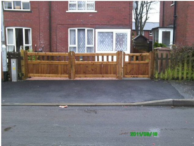
New dropped crossing and in-curtilage parking.
