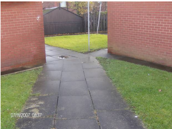
Path between bungalows before fencing
