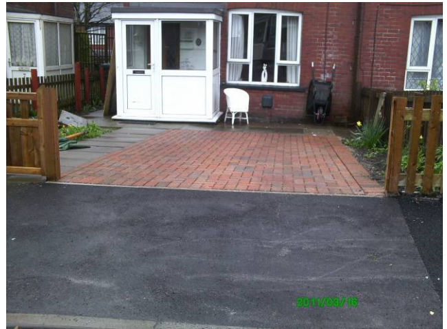
New driveway with block paving.
